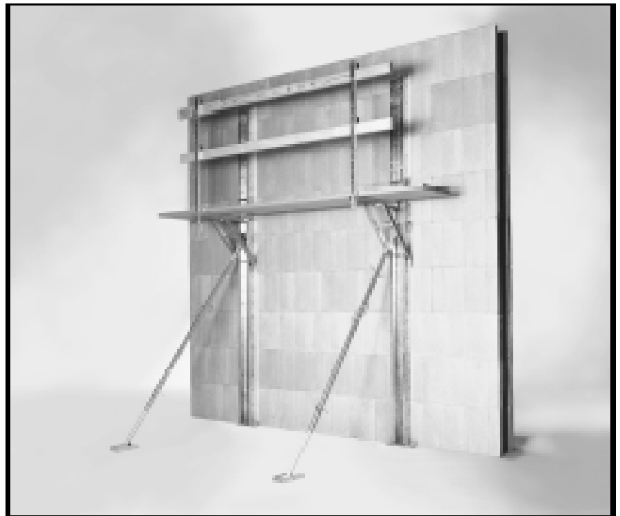
Third Course and Wall Alignment Installation
