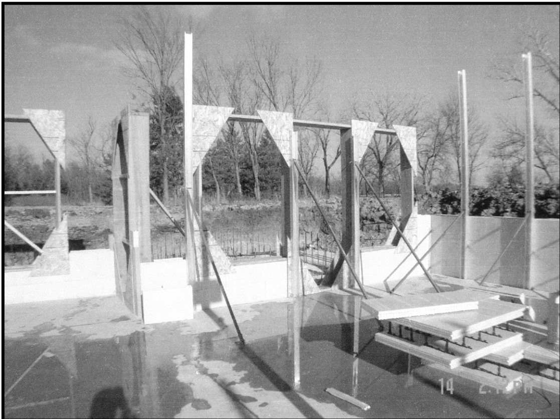
Second Course, Leveling and Wall Openings
